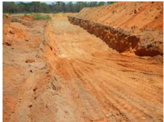
Next cell constructed and banded to prevent premature access
